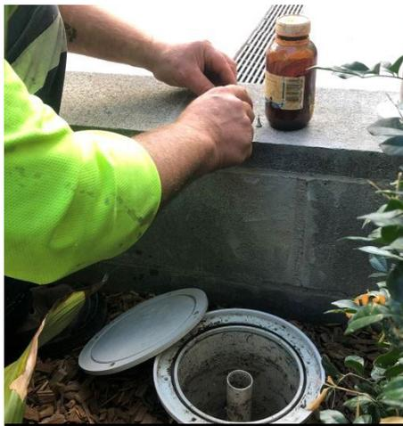
Using dye to assess connections within the catchment
