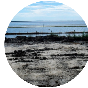
Figure 2. Active works underway - modified slope with sediment controls
