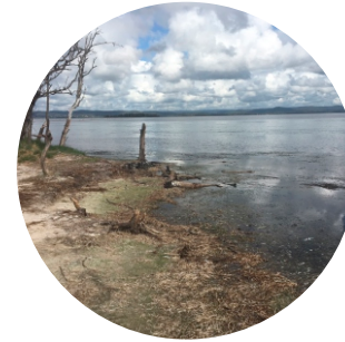
Figure 1. A modified and eroded foreshore.
