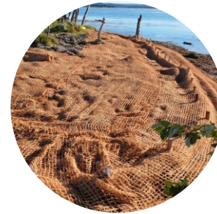
Figure 3. The road to recovery - passive rehabilitation - wrack mulching and coir mesh
