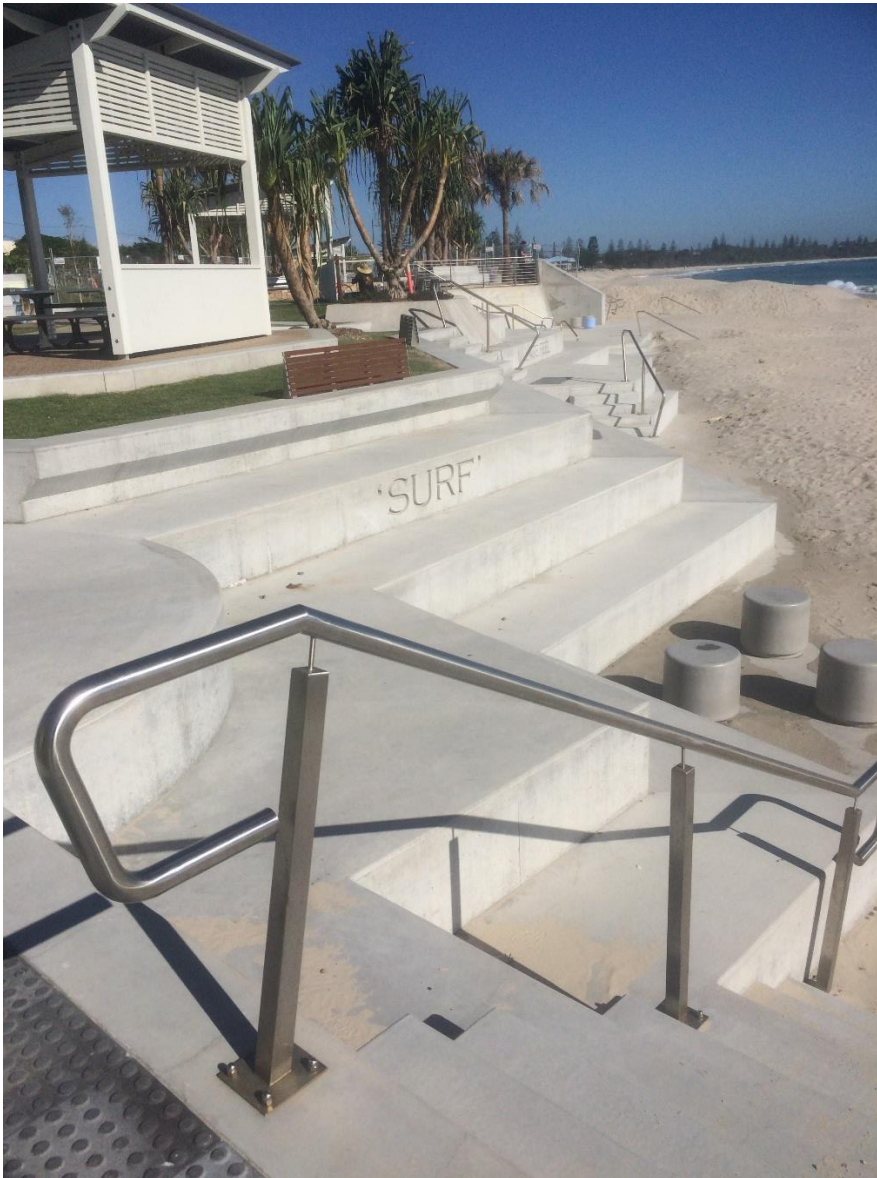
Figure 18: Recent stepped seawall installation at Kingscliff Beach (2018)
