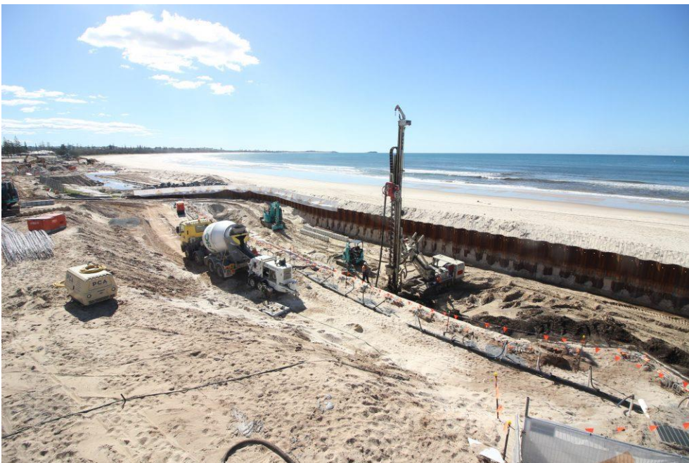
Figure 14: Installation of secant pile wall at Kingscliff Beach (Source: SEE Civil)
