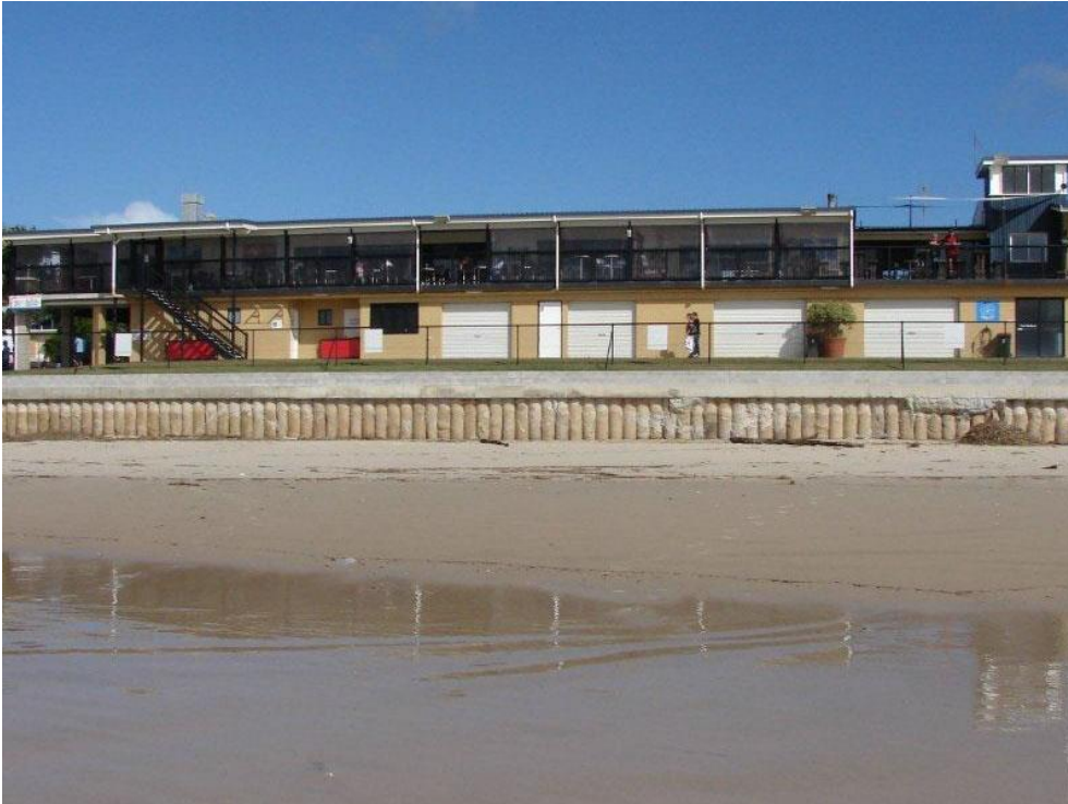
Figure 13: Secant pile wall with concrete capping beam installed in front of Cudgen Surf Club, Kingscliff (Source: ASP)
