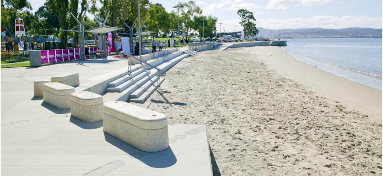
Figure 16: Stepped seawall at Sandy Bay, Hobart incorporating beach access steps
