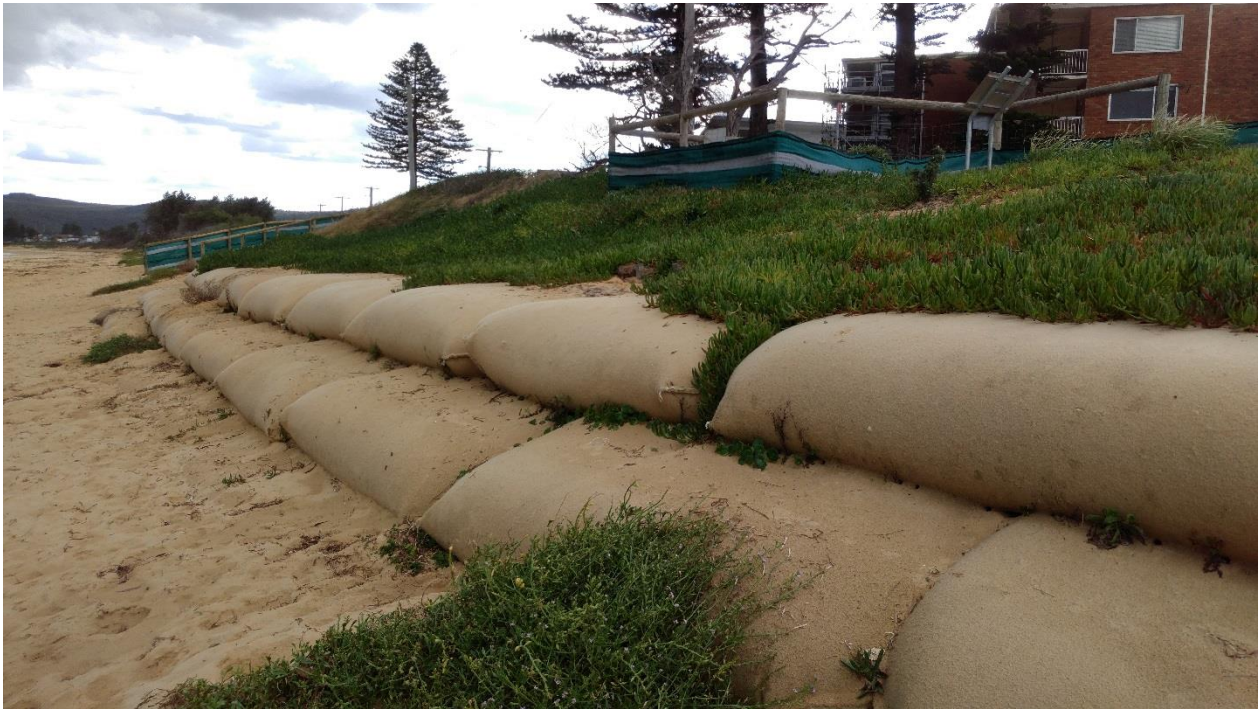
Figure 19: Geotextile container wall installed at Barrenjoey Road
