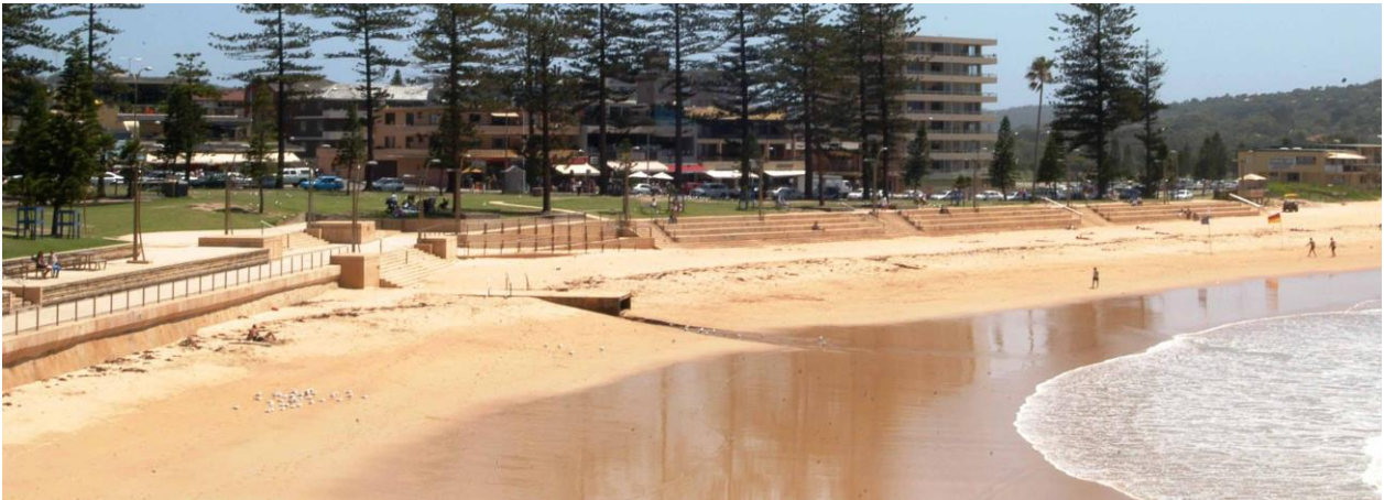
Figure 17: Stepped seawall at Dee Why Beach constructed in 1999, coloured to match natural colour of beach sand
