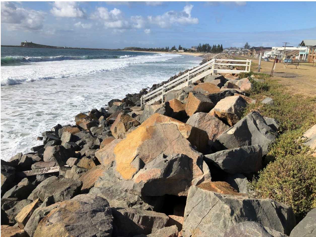
Figure 12: Seawall constructed from igneous rock at Stockton Beach, NSW
